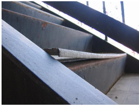
A stair tread in need of immediate repair. The unrepaired tread is a serious trip hazard on a busy stairwell.
