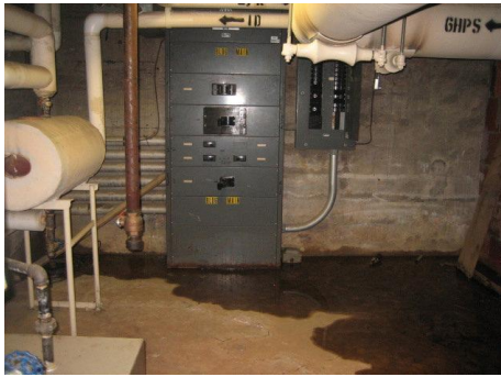
A water leak near a high voltage electrical panel has the potential to cause a deadly explosion.
