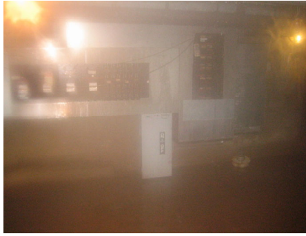
A steam leak in an electrical area could result in a power outage, along with other failures and damage.
