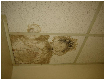
The stain indicates a leaking pipe in the ceiling. Such leaks can create the environment for growth of mold and mildew, some of which can be toxic.
